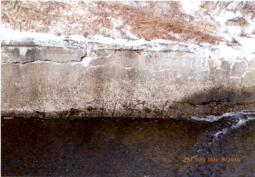
Photo 17 Dam ID# 188-0783 Woodward Lake Dam 01/08/2016 Concrete deterioration on the service spillway's left downstream training wall as observed from the service spillway's right side.
