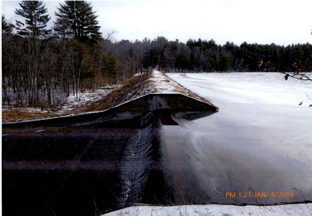
Photo 8 Dam ID# 188-0783 Woodward Lake Dam 01/08/2016 Service spillway, service spillway's right training wall, spillway discharge chute, and right embankment section as observed from the spillway's left side.
