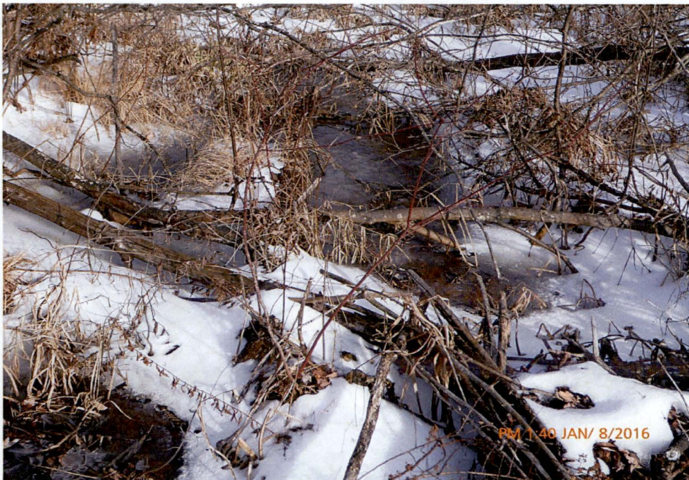
Photo 18 Dam ID# 188-0783 Woodward Lake Dam 01/08/2016 Ice observed at the right embankment's downstream toe. Could not determine if this was seepage of run-off from the embankment's toe.
