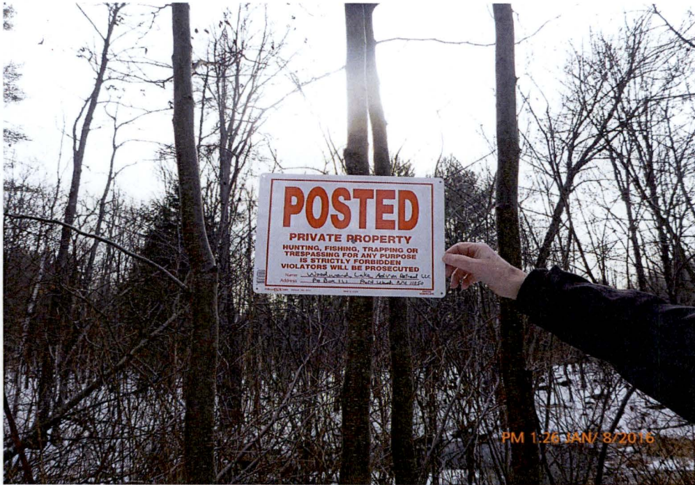
Photo 9 Dam ID# 188-0783 Woodward Lake Dam 01/08/2016 Posted sign on entrance path to the dam's right side.
